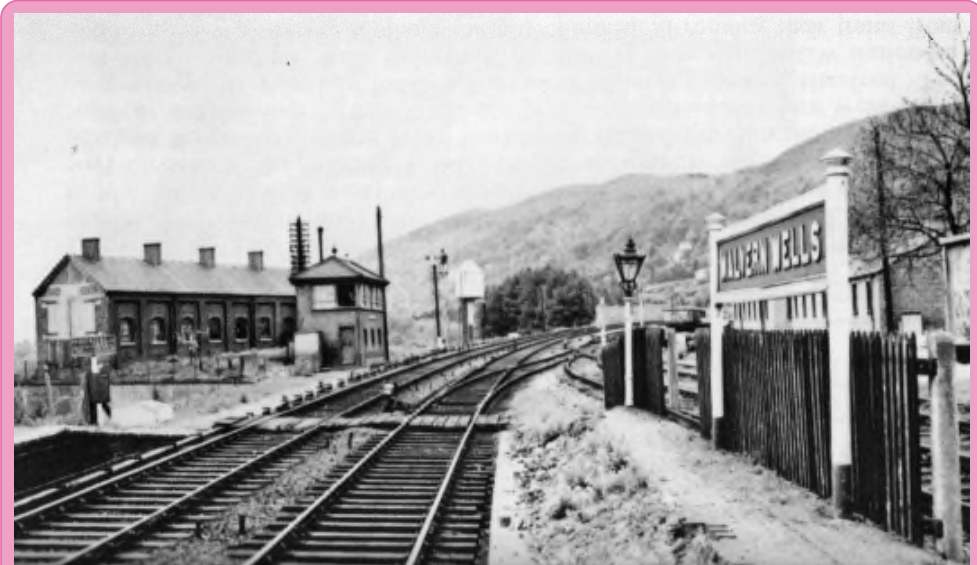
The water column, behind the signal, at Malvern Wells on the 1:80 climb up to the tunnel where “Top ‘em up Ted” would often stop for water giving a well-earned break from shovelling for the fireman
