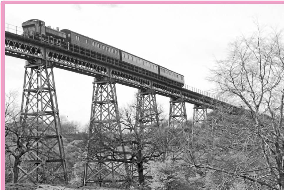
An ex-GWR Class 7400 Pannier Tank No. 7428 crosses Dowery Dell Viaduct on 19 April 1957 (Neville Stead Coll'n)
