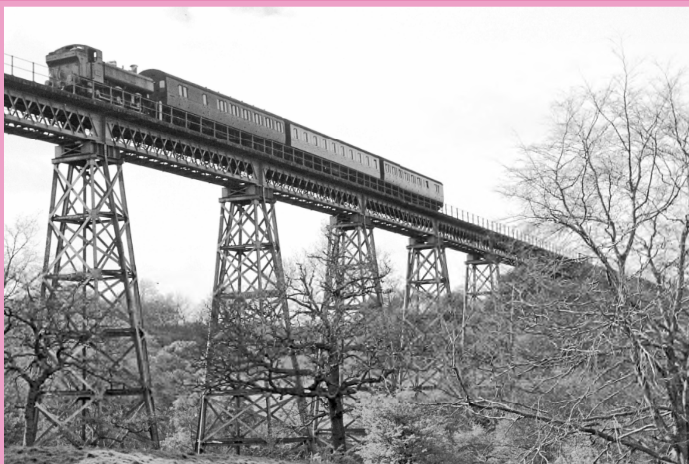
An ex-GWR Class 7400 Pannier Tank No. 7428 crosses Dowery Dell Viaduct on 19 April 1957
