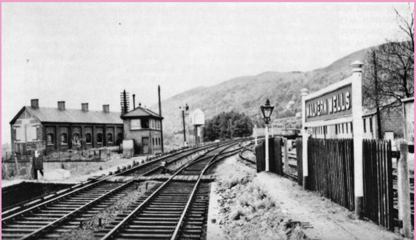
The water column, behind the signal, at Malvern Wells on the 1:80 climb up to the tunnel where "Top 'em up Ted" would often stop for water giving a well-earned break from shovelling for the fireman
