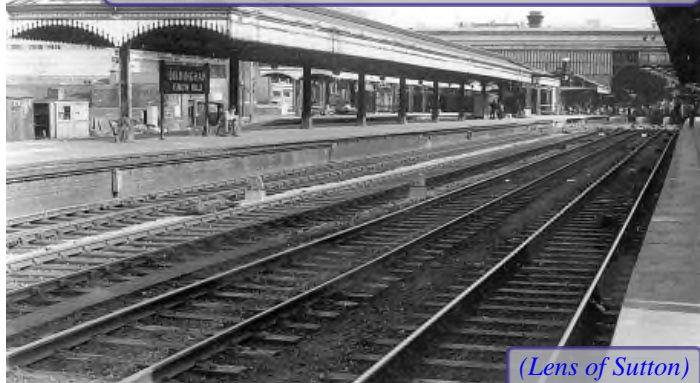
A view from the far end of platform 6 shows the 4 tracks between the main platforms
