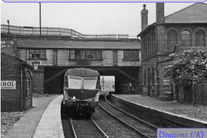
Dudley Port Low Level (1950) with the high level platforms above. The GWR railcar is passing through without stopping.
