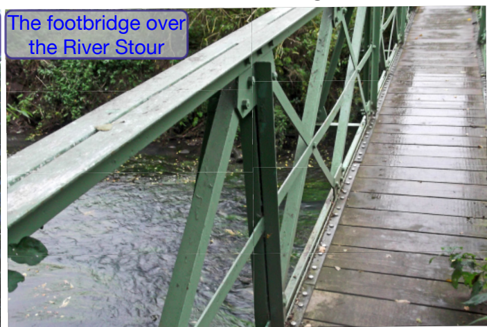
Stambermill Viaduct and the footbridge over the River Stour
