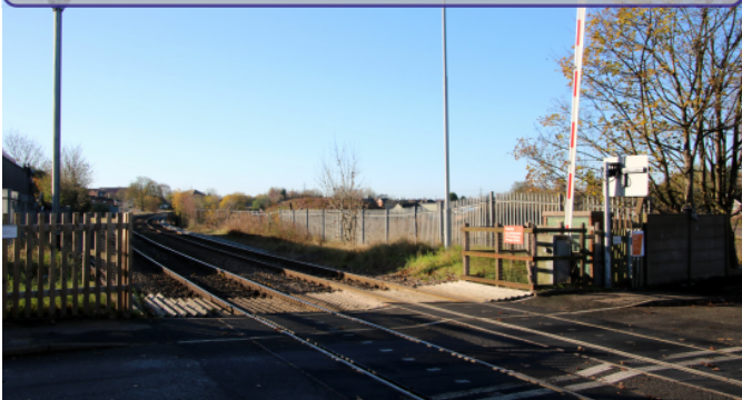
Station Road, Langley Green, the site of the original Oldbury & Langley Green station
