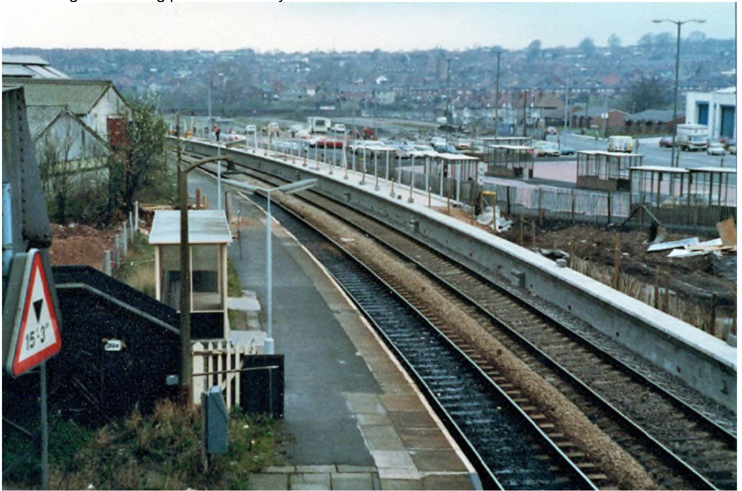
Rebuilding work taking place at Cradley Heath station from 1981 to 1983.
