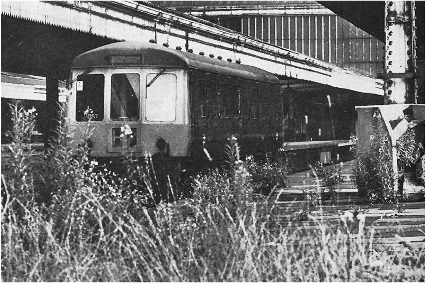
Birmingham Snow Hill and Wolverhampton Low Level both closed in 1972, and both looked a sorry sight a year before closure.
